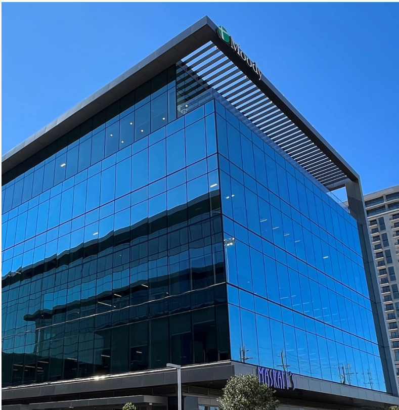
Village Towers, Houston, TX, USA – Photo © Steve Versland | Example of Façade Visual Harmonization
