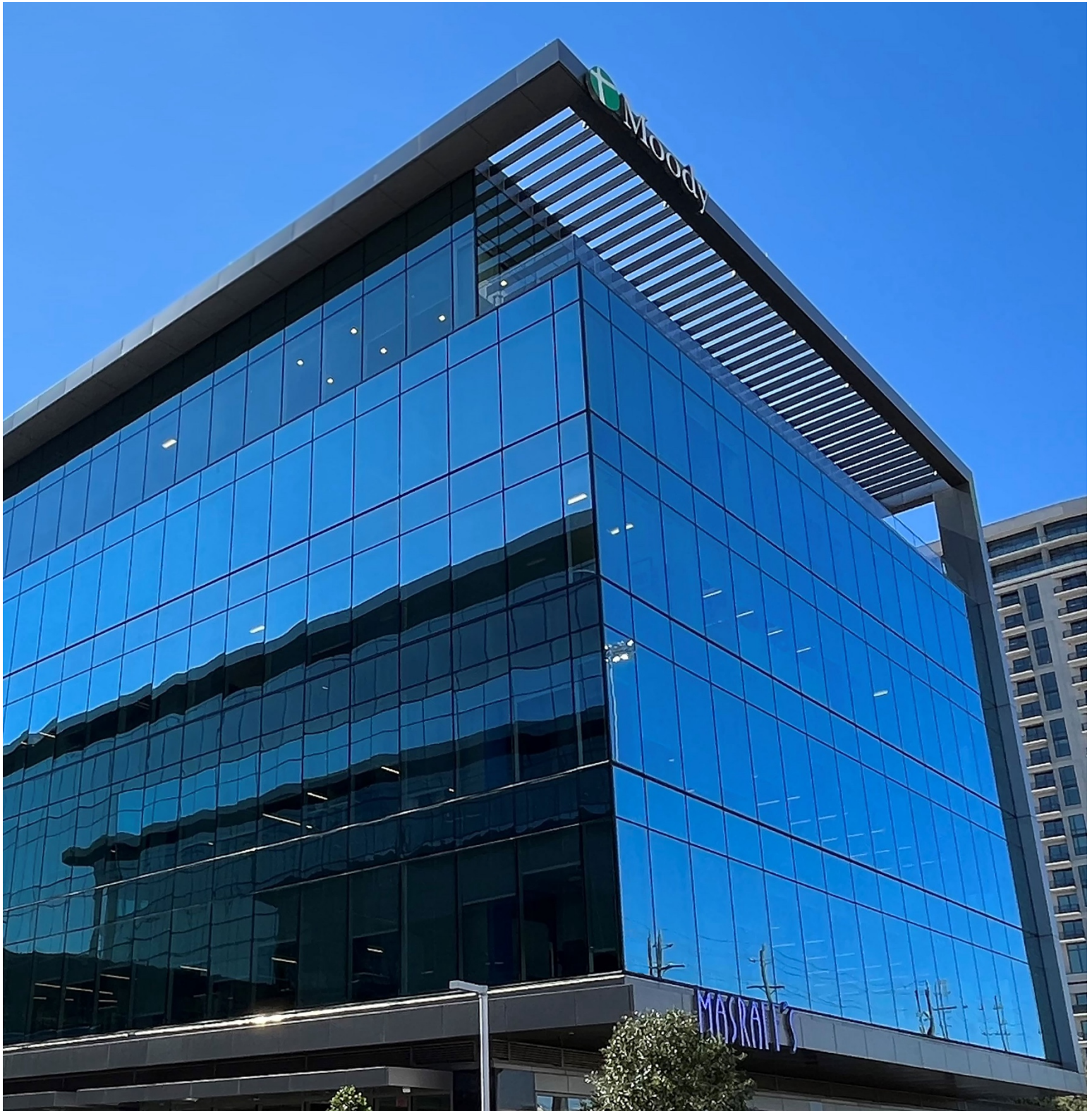
Village Towers, Houston, TX, USA – Photo © Steve Versland
